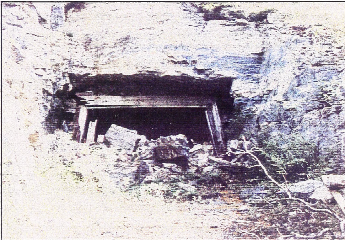
South or lower end of Cape Horn tunnel. This is the least disturbed of any of the tunnel entrances on the Miocene ditch.
