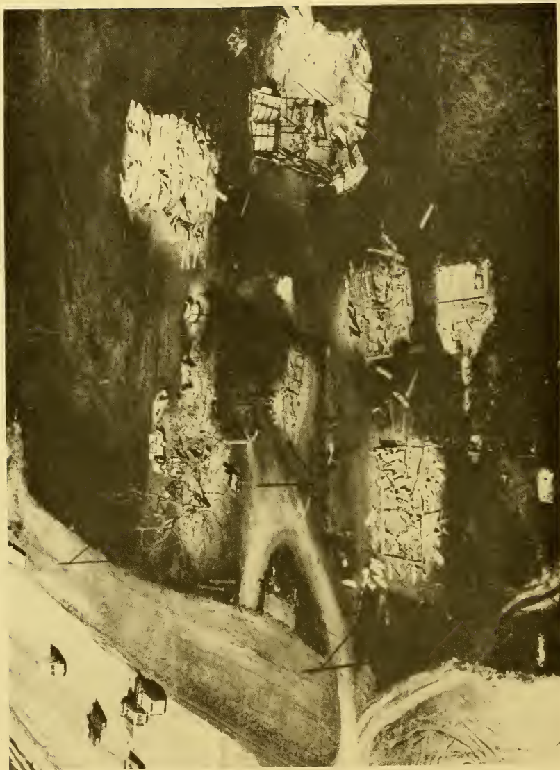
Figure 4. An aerial view of the farmhouses and other outbuildings destroyed.
